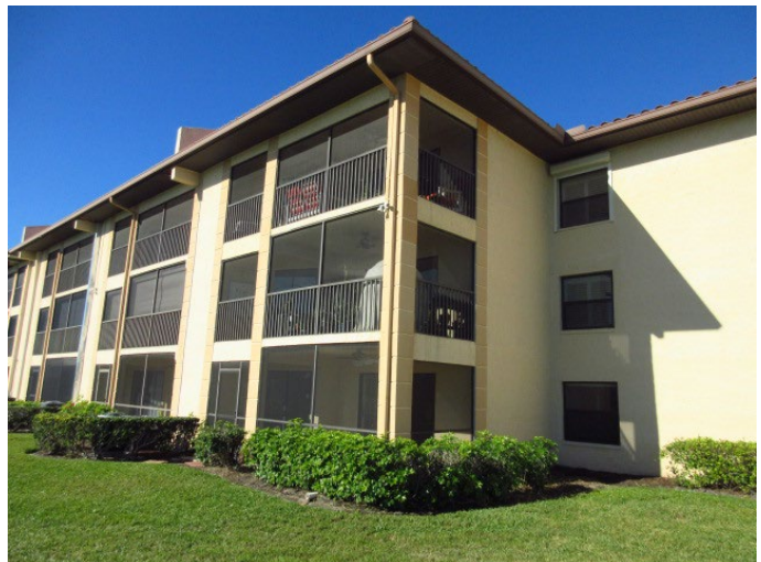
VIEW OF BUILDING EXTERIOR FINISHES
