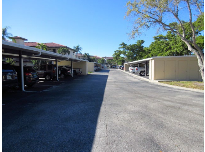
GENERAL VIEW OF PARKING AND PAVEMENT
