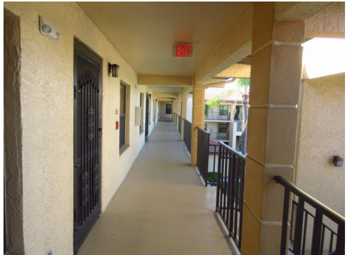
VIEW OF ELEVATED WALKWAY
