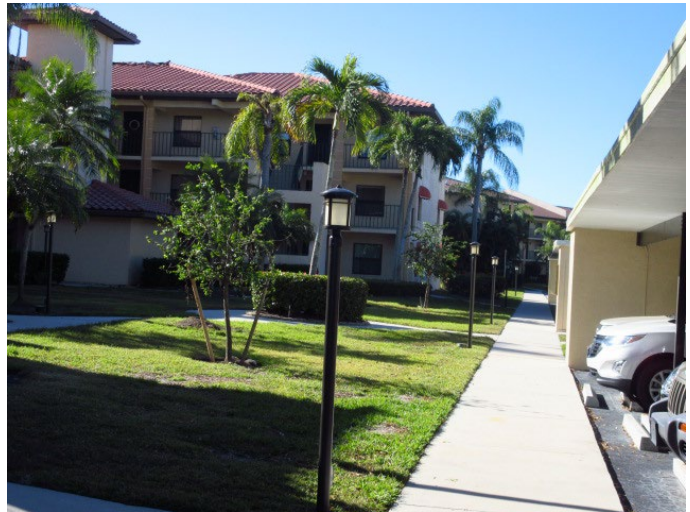
VIEW OF SITE LIGHTING
