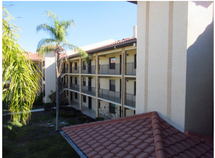
VIEW OF ROOF COVERING
