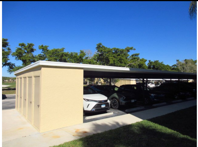
VIEW OF STORAGE UNITS AT CARPORT
