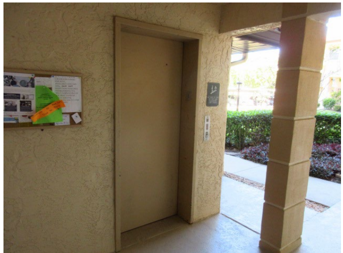
VIEW OF ELEVATOR LOBBY
