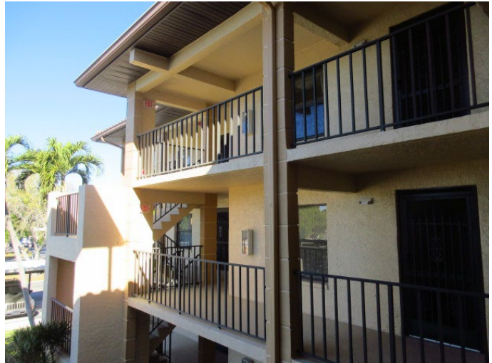
GENERAL VIEW OF BUILDING EXTERIOR FINISHES
