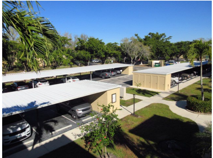
VIEW OF CARPORTS
