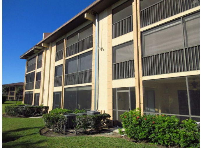
GENERAL VIEW OF BUILDING EXTERIOR FINISHES
