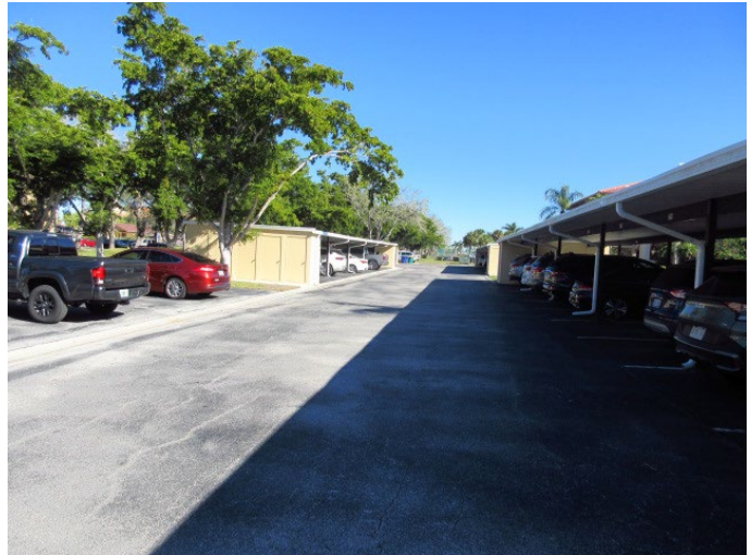
GENERAL VIEW OF PARKING AND PAVEMENT
