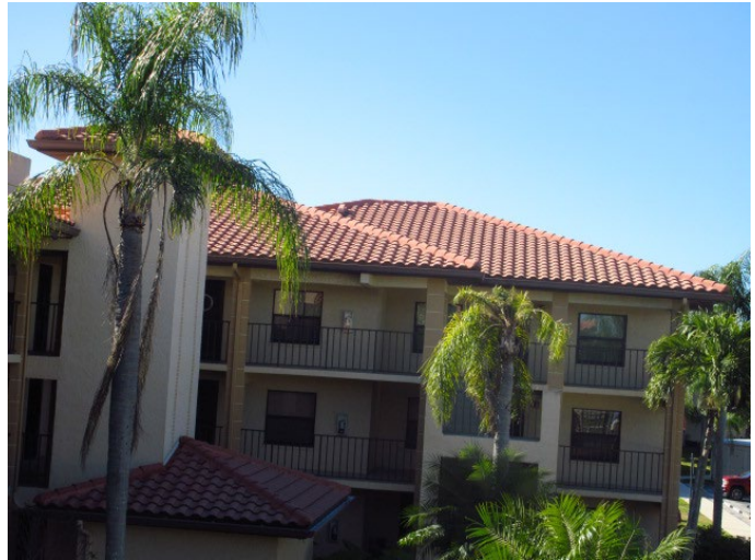
VIEW OF ROOF COVERING
