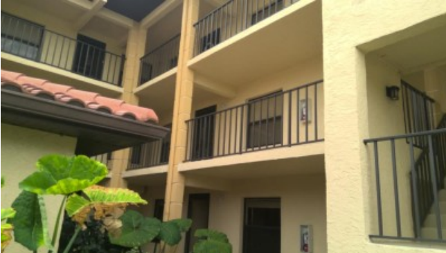
Building Front Photo
