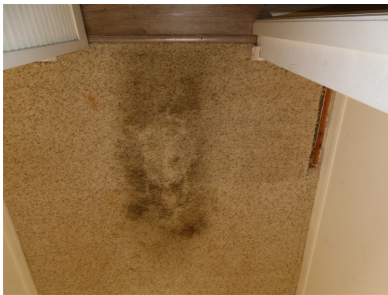
2.0 Item 1 (Picture) Master bathroom closet
